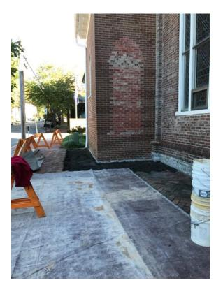
The work on waterproofing the church foundation continues along Washington Street. When finished, the city will replace the lumpy sidewalk on that side of the church.
